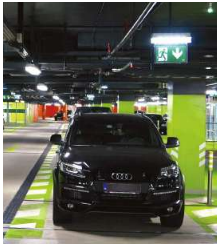
Parking Garage Area Emergency Lighting Application
