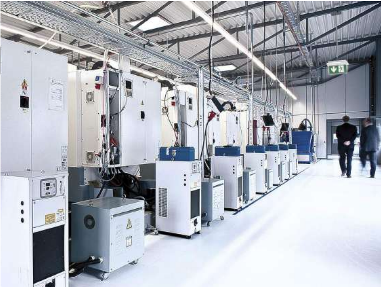
Industrial Area Emergency Lighting Application
