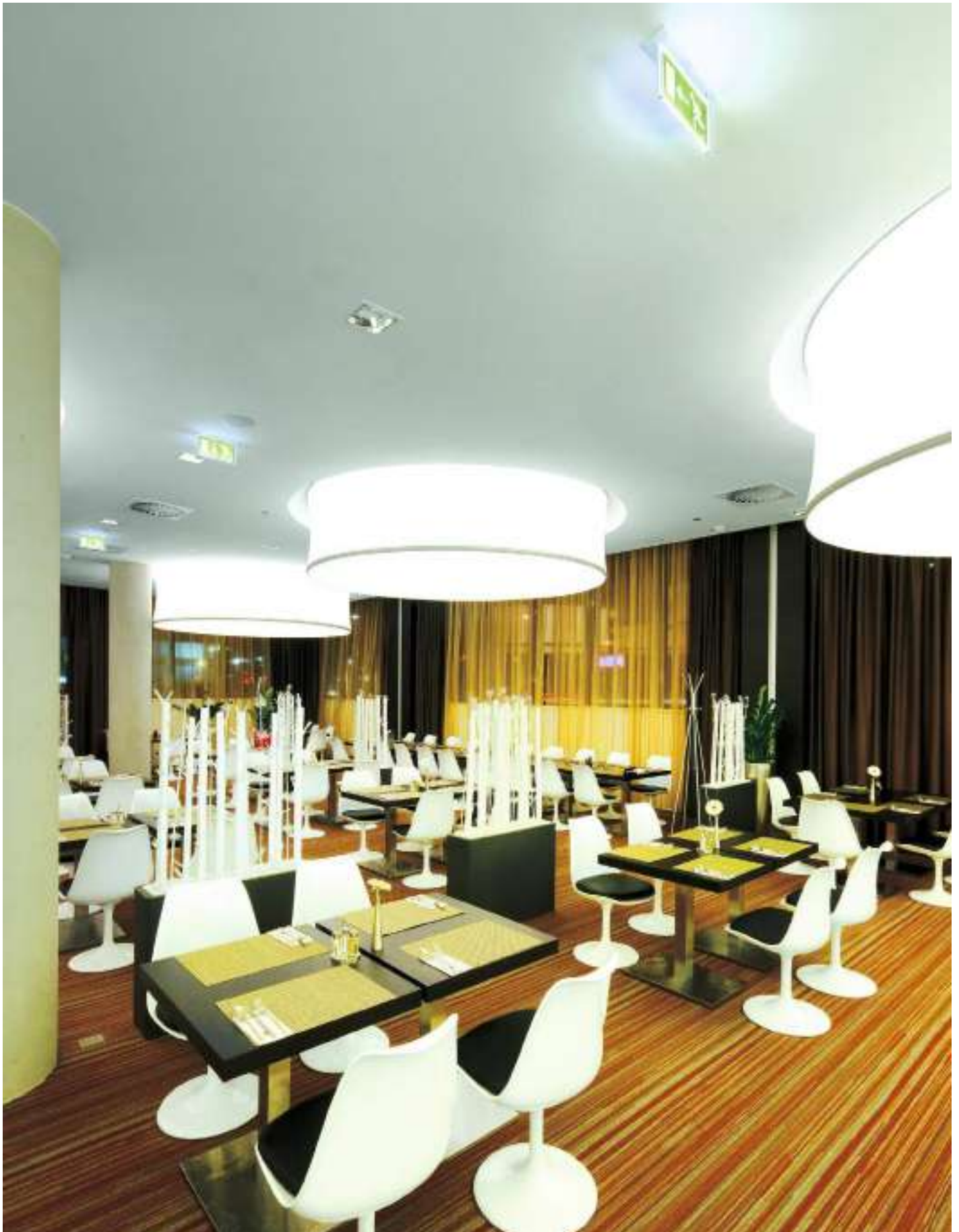
Hotel restaurant area emergency lighting application
