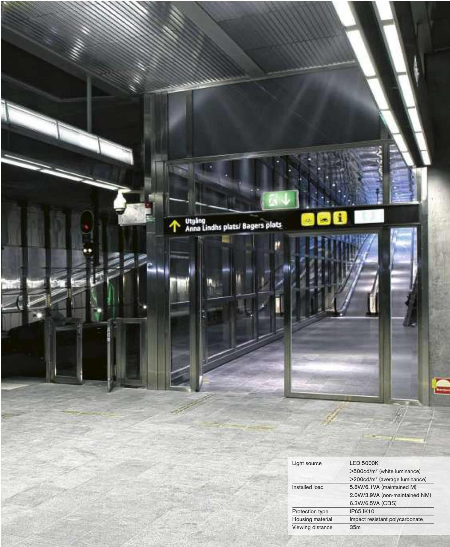
Train station area emergency lighting application
