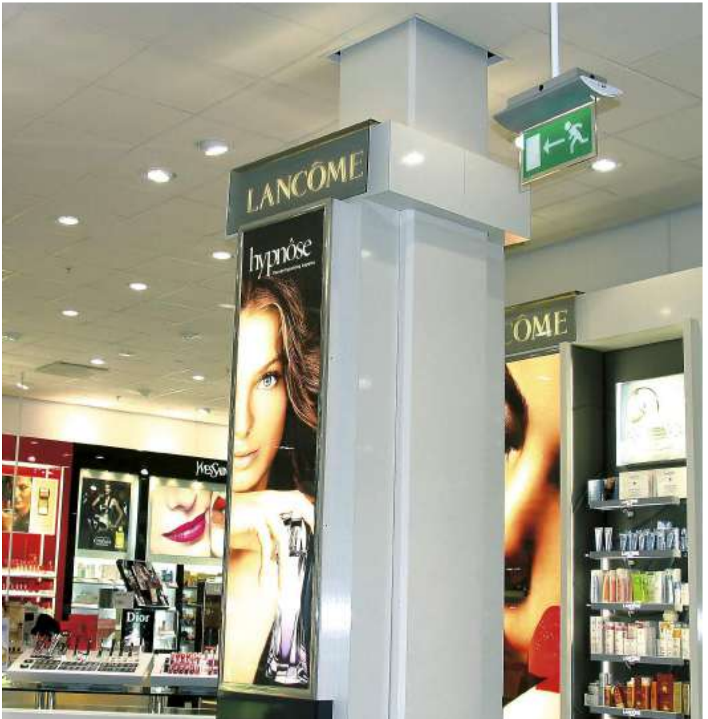
Shopping area emergency lighting application
