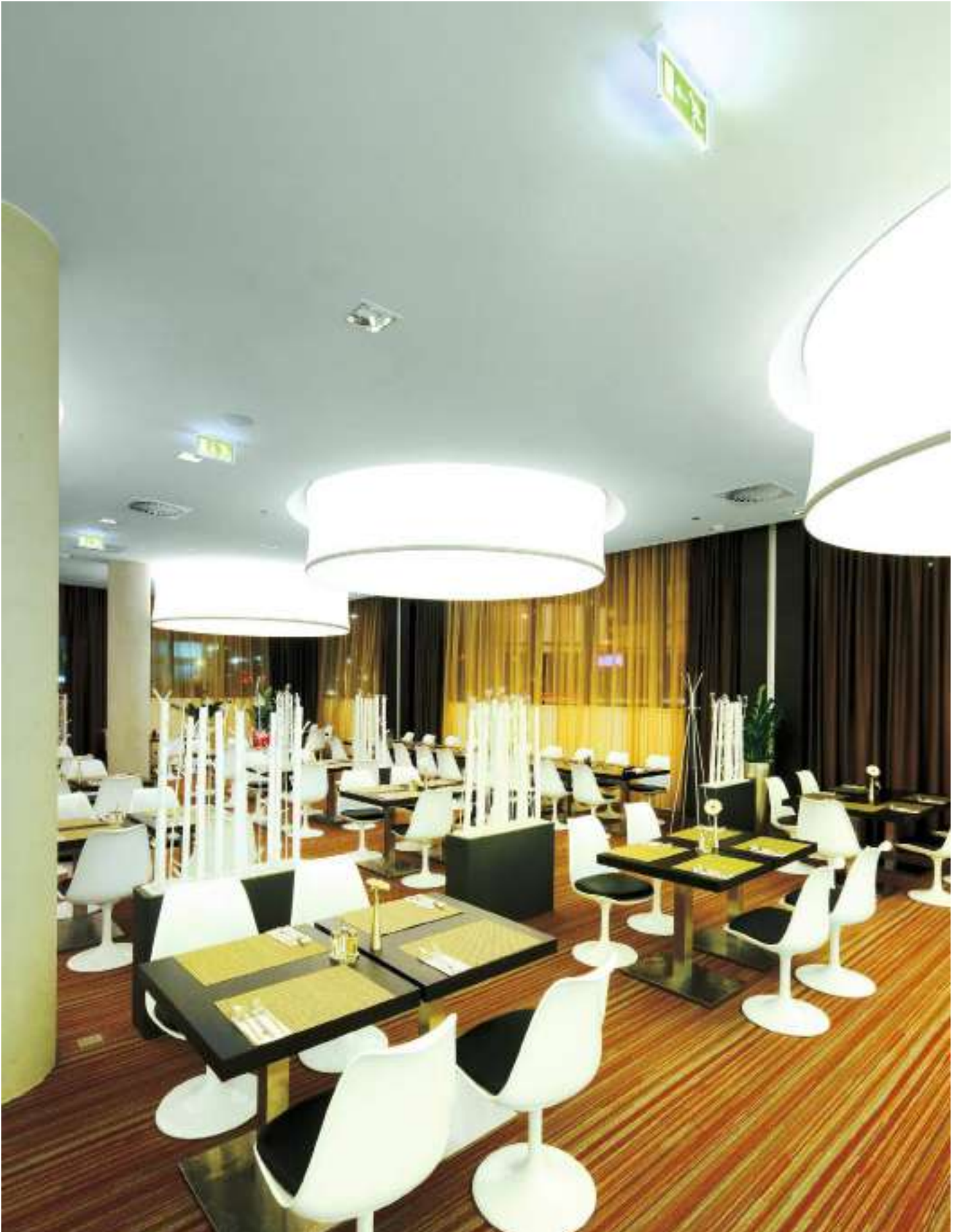
Hotel restaurant area emergency lighting application
